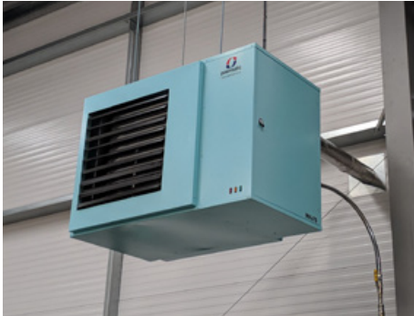
New Warm Air Heaters supplied & installed
